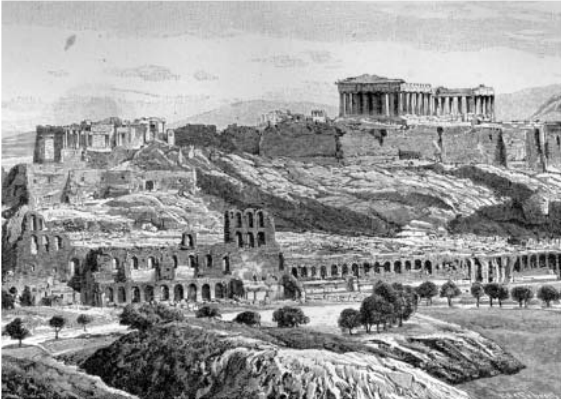
Fig. 7.35. General view of the ruins of the Athenian Acropolis from its southern side. Its XIX century condition. Taken from [304], Volume 1, page 160.
