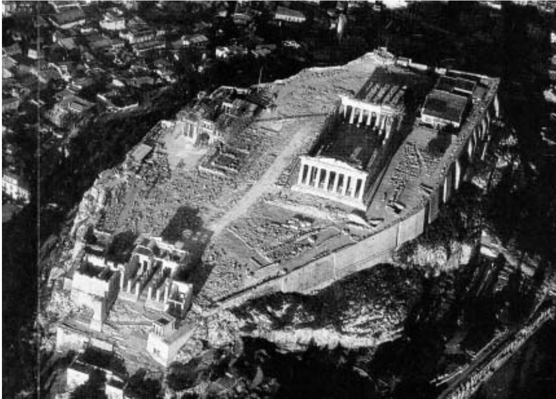
Fig. 7.45. A modern view overlooking the Acropolis. It is plainly observable that the “ancient” buildings left intact by the restorers comprise a visible minority of the entire architectural group that had occupied the entire top of the rock in the Ottoman epoch. Apparently, most of the buildings were too obviously Christian, dating from the XV-XVI centuries. This is why they had to be demolished “so that the ancient landscape could be restored”. Taken from [198], pages 100-101.
