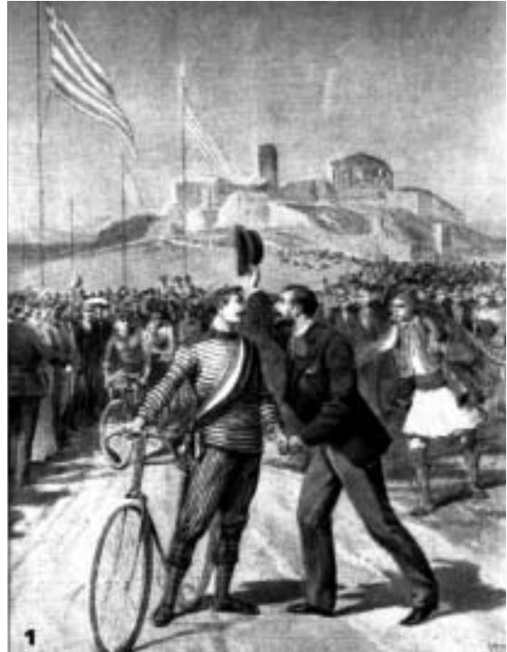
Fig. 7.44. A picture taken from 1896 depicting the subsequently demolished Ottoman tower on the Acropolis. It was taller than the Parthenon . Taken from [340], page 40.
