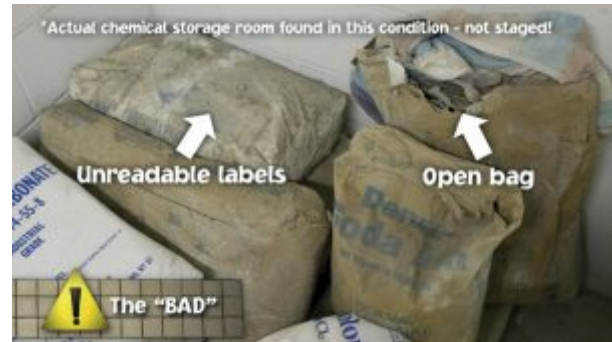
Figure 3. Example of improper chemical storage
