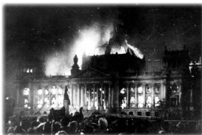
Figure 10.3: The burning Reichstag. The Reichstag building is a historical edifice in Berlin, Germany, constructed to house the Imperial Diet (German: Reichstag), of the German Empire. It was opened in 1894 and housed the Diet until 1933, when it was severely damaged after it was set on fire.
